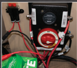
DUAL BATTERY HARNESS W/SWITCH
